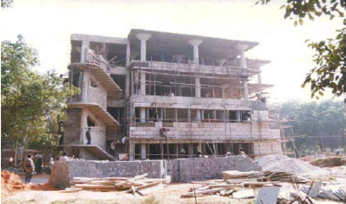
4 storey building constructed using flyash bricks at Indian Institute of Technology, New Delhi
