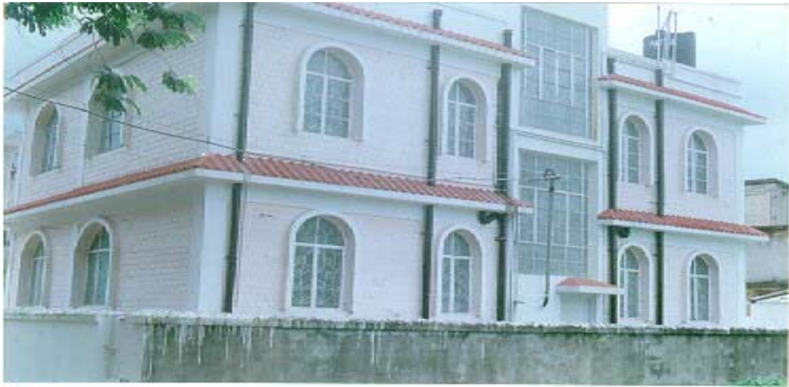
Building constructed using fly ash bricks at Calcutta, West Bengal
