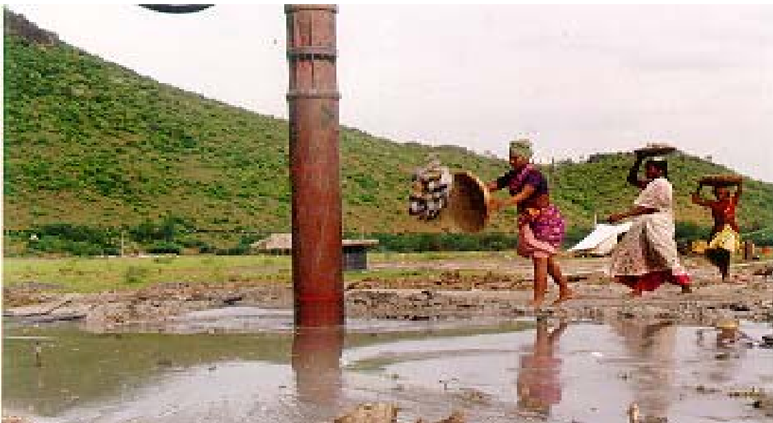
Densification by Vibroflotation, Vijaywada Thermal Power Station, Andhra Pradesh
