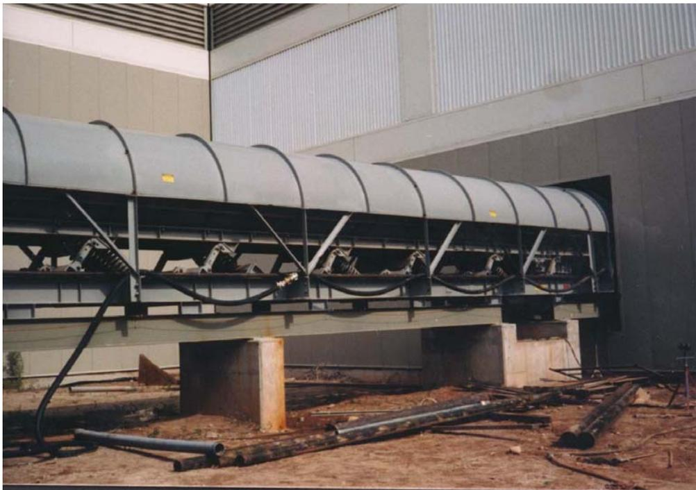
**Figure 9 Hooded Vibratory Conveyor in Mass Burn Facility**
