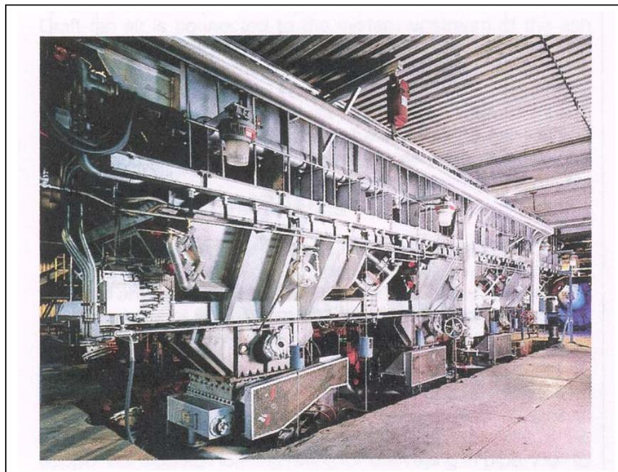
Figure 2: A view of Dry Bottom Ash Hopper (PAX™ Pneumatic Ash Extractor) installed at Florida Power Corp., Crystal River Unit 1.
