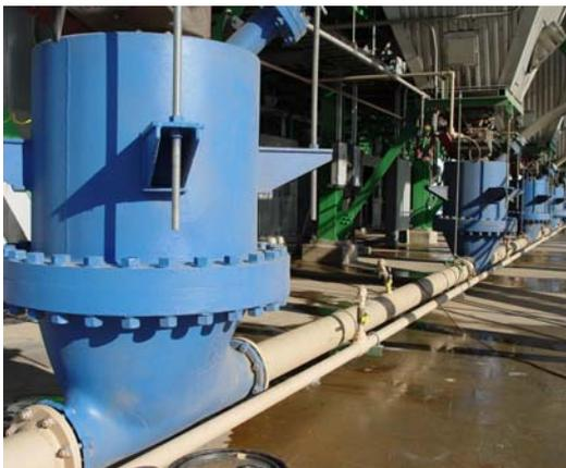
Figure 15. Typical MultiDAC™ Dense Phase Transmitter
