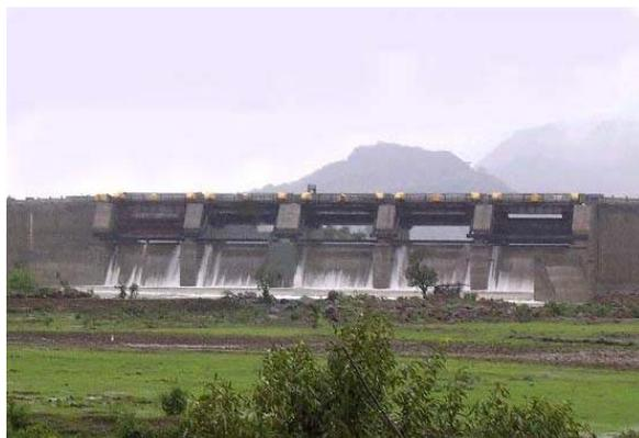
Upper dam of Ghatghar Pumped Storage Scheme constructed with RCC ( 65% replacement of cement with fly ash)
